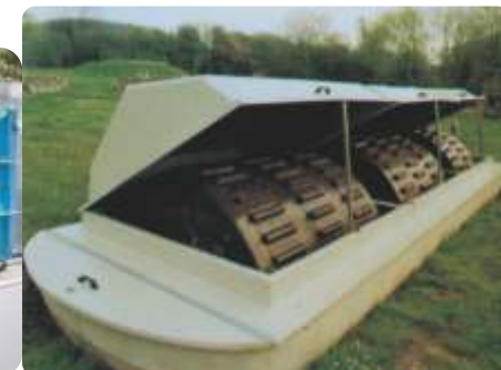
INDION New Generation Packaged Sewage Treatment Plant (NGPSTP)
